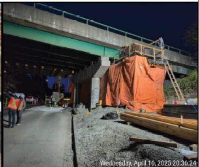
Figure 5: Heating and Hoarding for Concrete Curing
