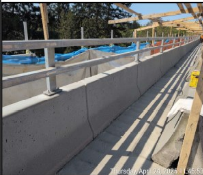
Figure 4: Installation of South Bridge Railing
