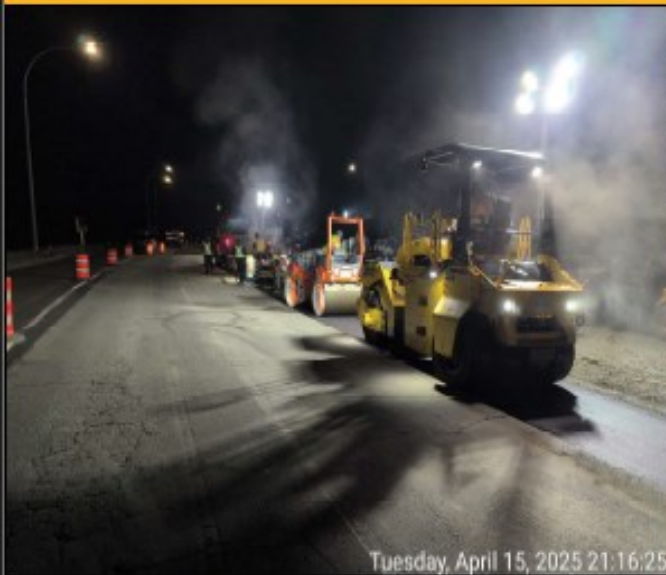
Figure 2: Highway 1 Shoulder Paving
