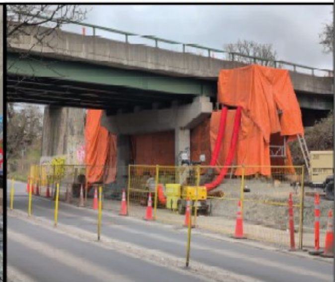
Figure 5: Heating and Hoarding for Concrete Curing
