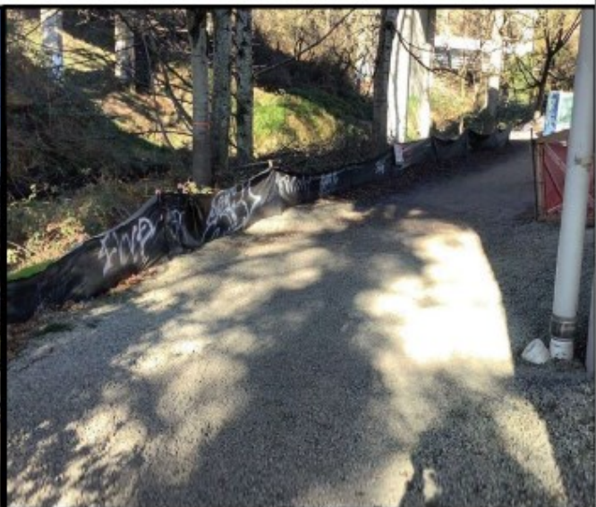
Figure 5: Silt Fencing Along Multi-Use Path
