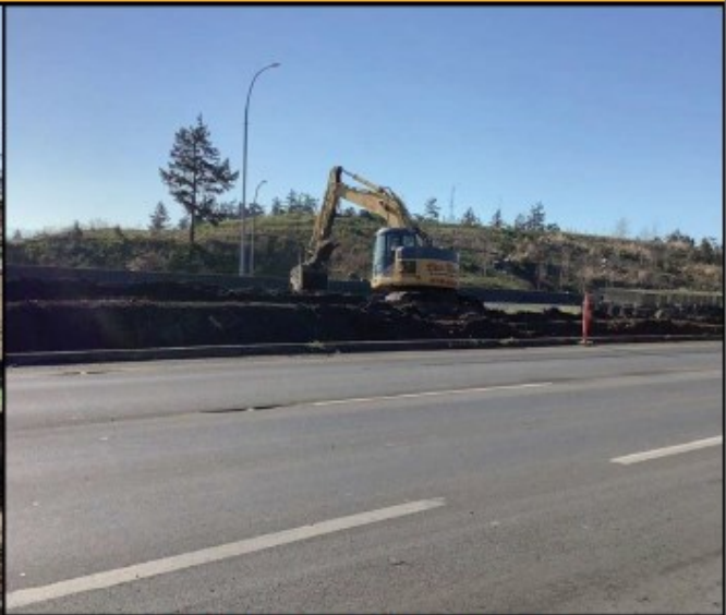
Figure 3: Works Along West Median on Highway 1
