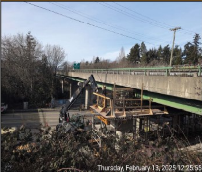
Figure 2: Work Along North Bridge Bent
