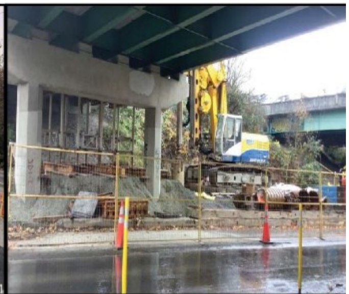
Figure 5: North Bridge Pile Installation
